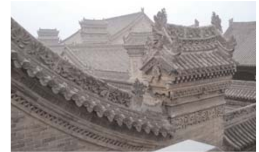
view over roof tops
